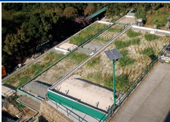
Aquatic vegetation growing in the new Constructed Wetland Wastewater Treatment System.
