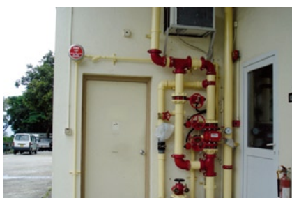
New fire services sprinkler system installed in the Conservation Building.
