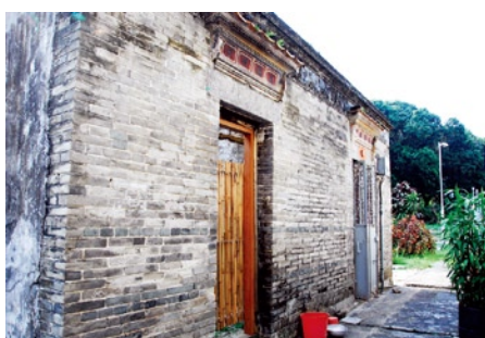
A simple bamboo door constructed by our Facilities Department to prevent access to the bat colony in a Lam Tsuen village house.
