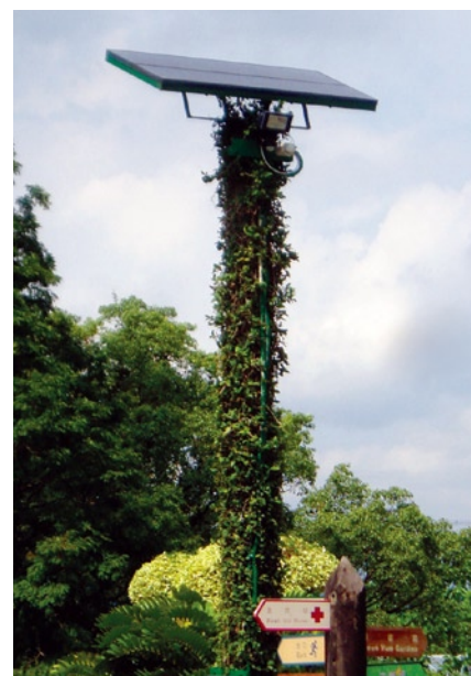
One of the solar-powered motion-sensing street light posts in KFBG.
