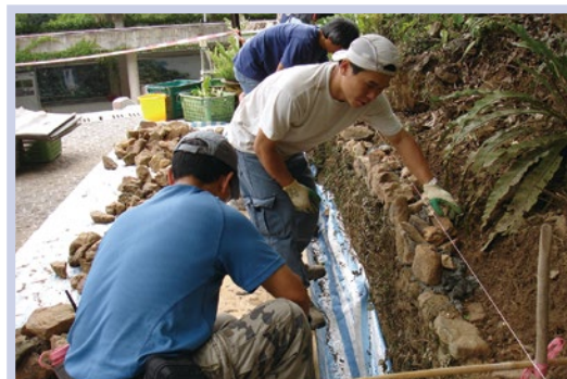
Staff constructing a planter wall on the sloping bank beside the Plaza (May 2011).
