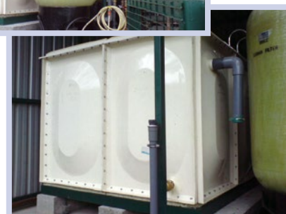
An industrial capacity sedimentation filter in KFBG to filter stream water.
