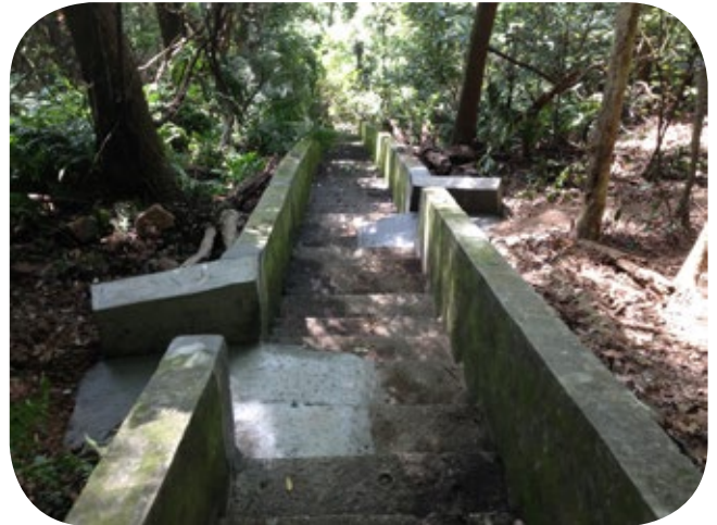
Animal friendly engineering along the Woodland Trail allows trapped animals to escape from the deep drainage channel
