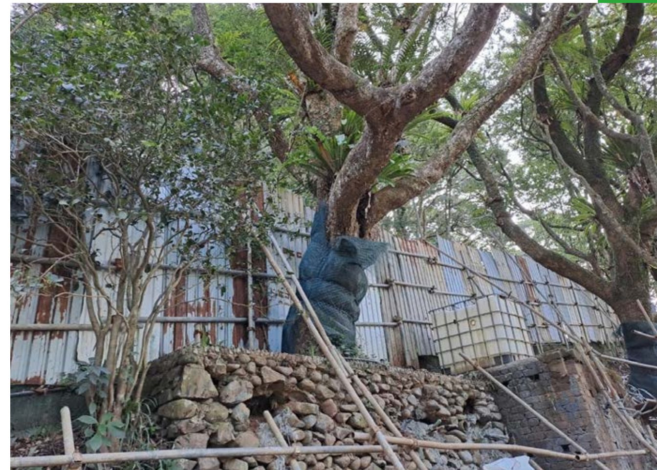
Existing tree trunk wrapped with erosion control mat
