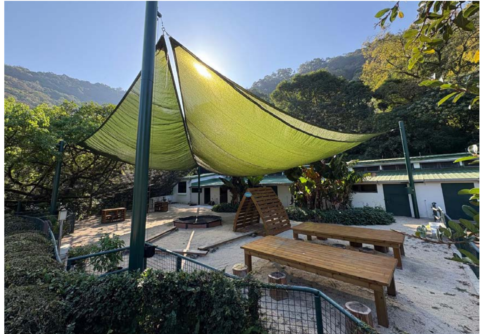
Installation of shading net in the outdoor play area
