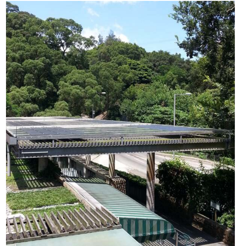
Mat type PV panels at Reception 接待處新造地墊式太陽能板
