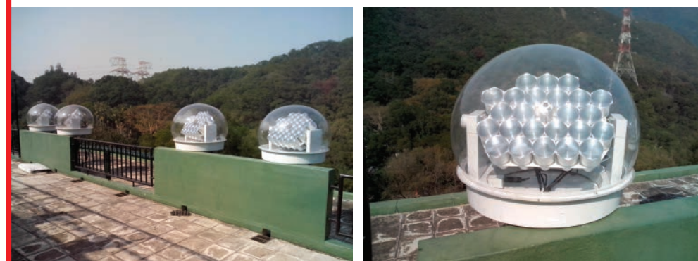
Installed new lens & optical fibre transmission devices at Education office 加裝太陽光纖導入器於教育部辦公室
